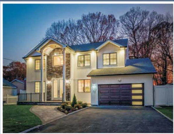
West Hempstead New Construction
